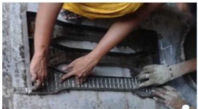
Placing mesh in the mould
