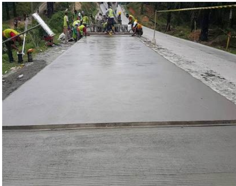
Figure 2. Rigid Pavement Constructions
