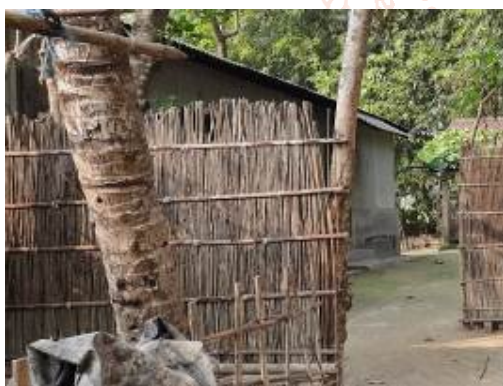
Fig.4 Jute sticks used as fencing material
