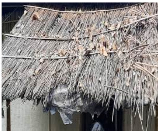
Fig.6 Jute sticks used as thatching material
