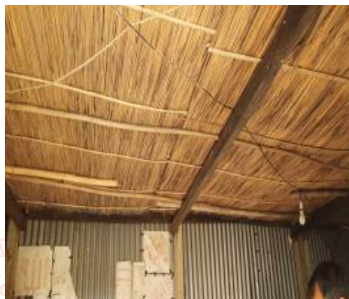
Fig.5 Jute sticks used as ceiling material
