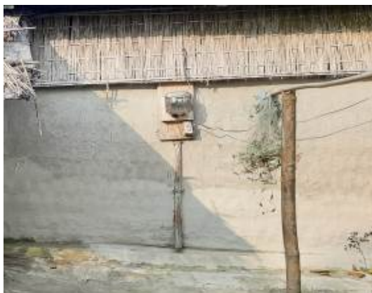
Fig.3b. Jute sticks used as wall with mud and cow dung
