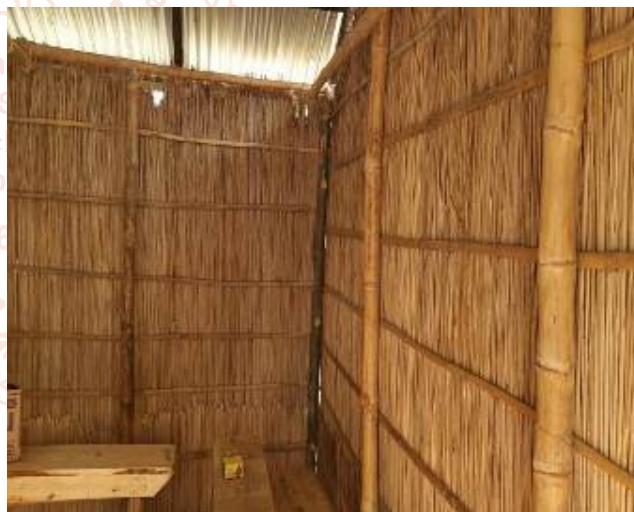
Fig.3a. Jute sticks used as wall
