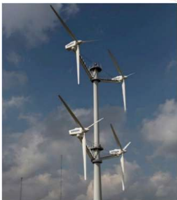
Figure 9: A multi-rotor wind turbine [10].
