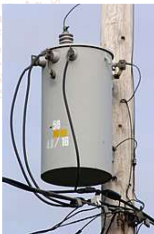
Figure 6: A pole-mounted distribution transformer [6].
