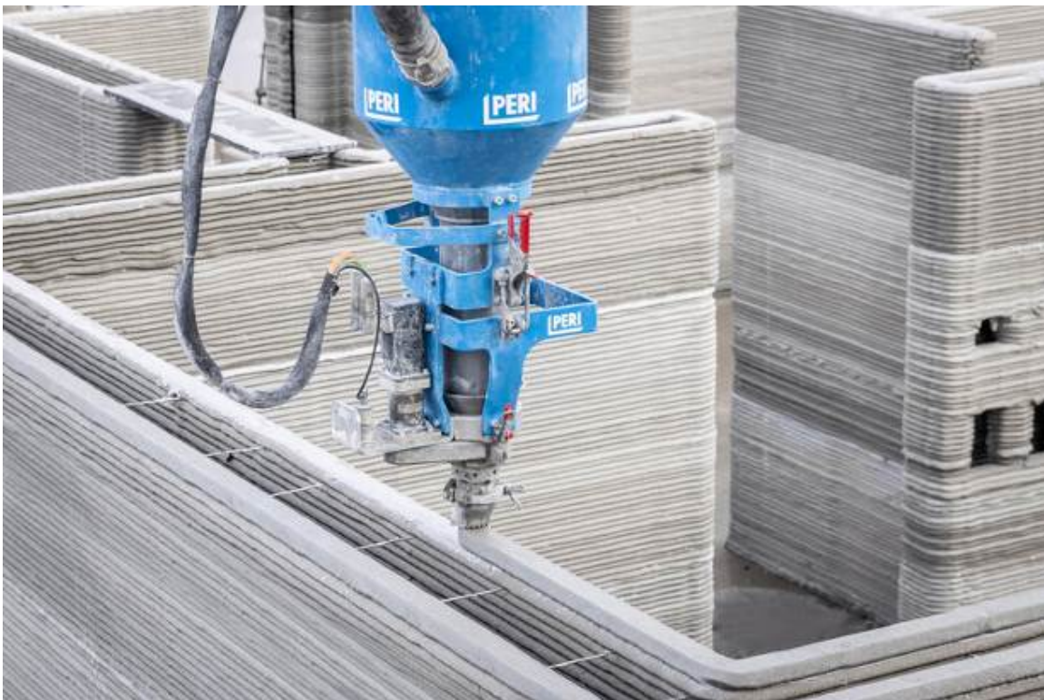
Figure 8 A building construction using 3D printing [10].
