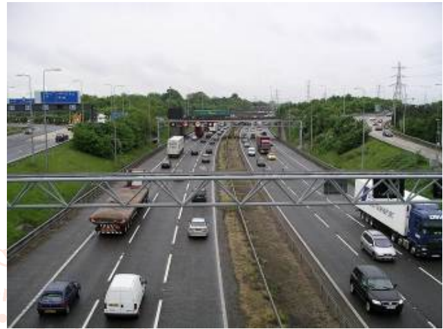
Figure 4 Active traffic management.
