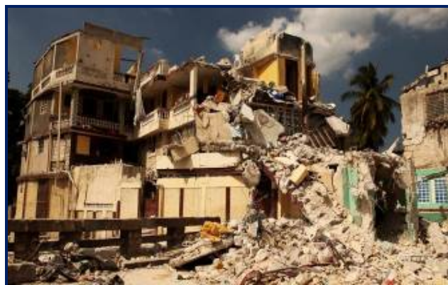
Fig. 2: Building Collapse due to Earthquake (Source: Earthquake in Turkey) [26]
