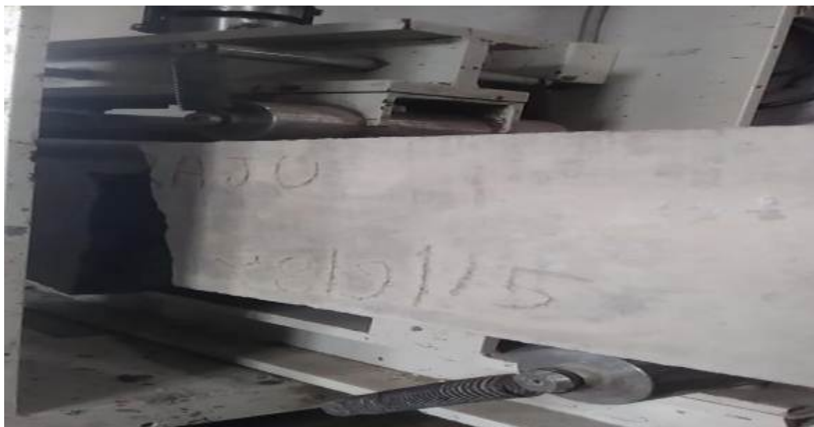
Figure No. 2.6: - BEAM CRACK PATTERN
