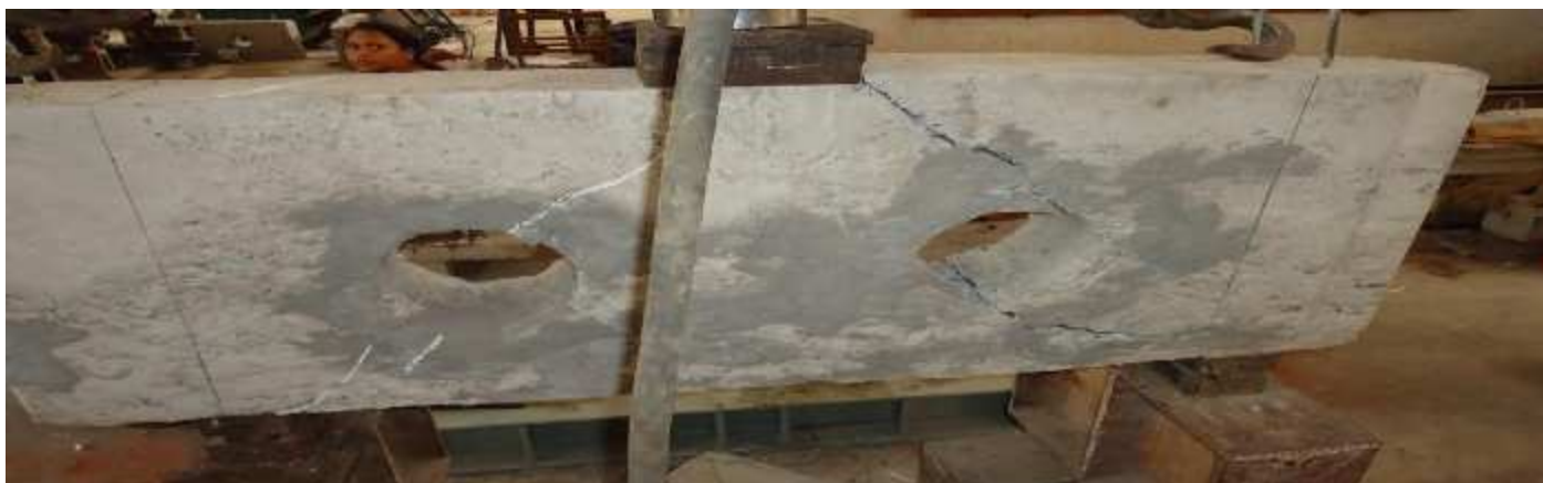
FIG. SPECIMEN SHOWING THE CRACK PATTERN (BACK)
