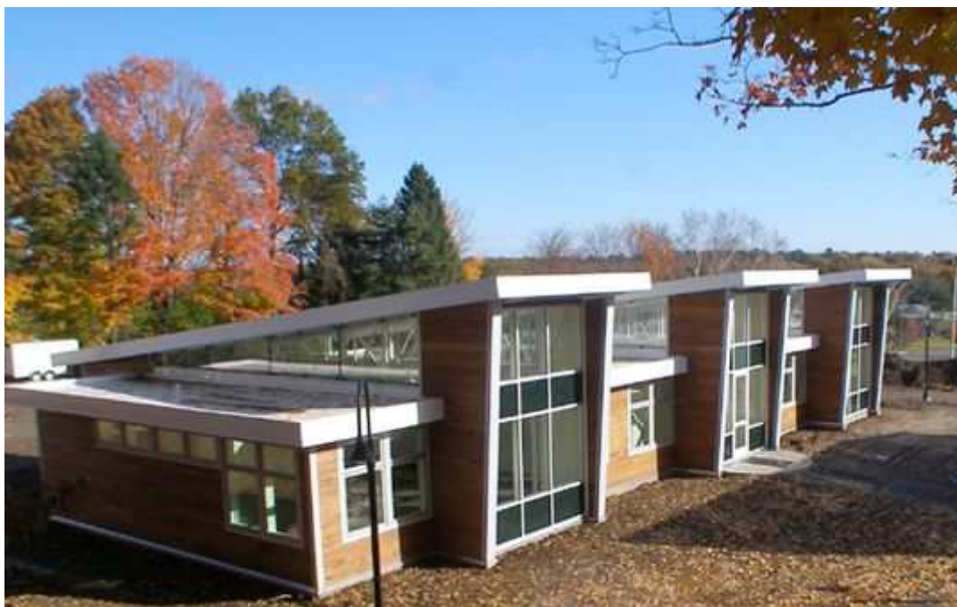
Fig.8 Eco-friendly Prefabricated Construction
