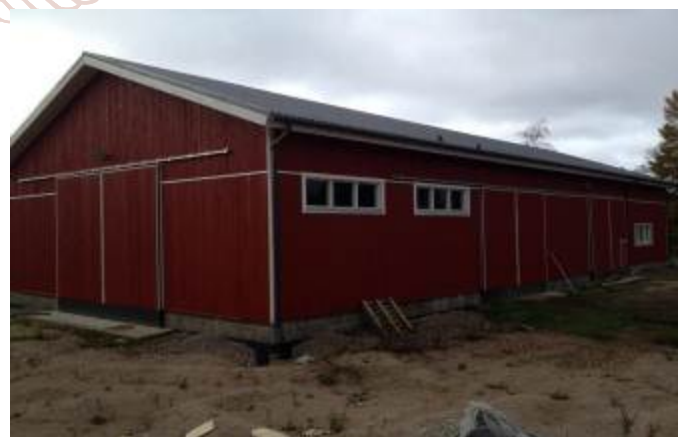
Figure 1 outside view of the building
