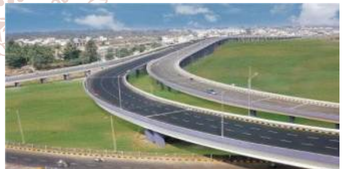
Figure 1.1 Road over Bridge
