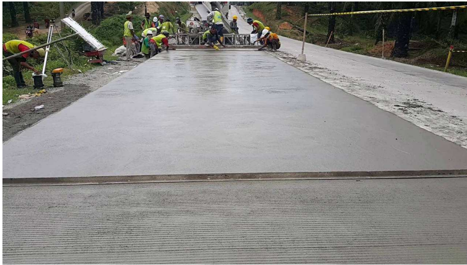
Figure 1.2 Rigid pavement construction
