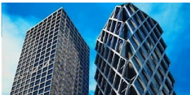
Figure 1.2 Conventional structure and Diagrid structure.
