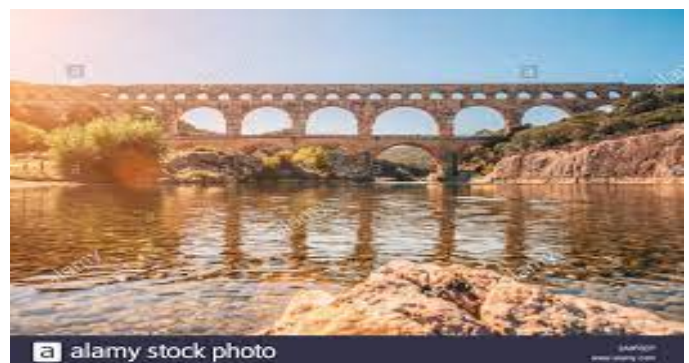
Fig 1.1 View of Ancient Bridge
