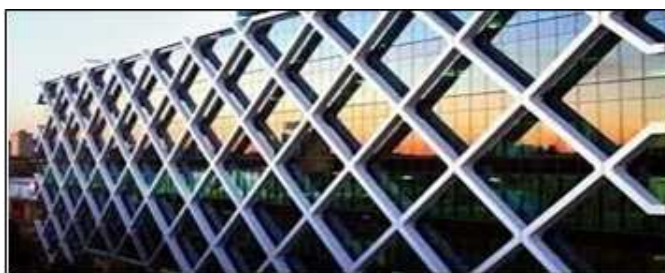
Fig 1 Steel diagrid structure
