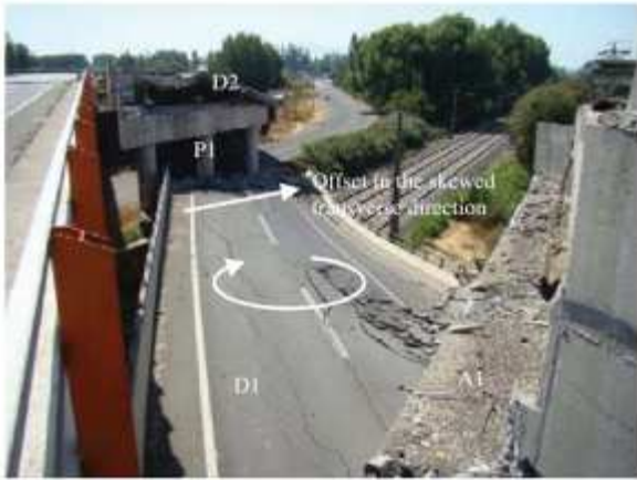
a) Hospital Overpass Bridge Collapse b) Collapse of Miraflores Overpass Figure 1.1 Failure of bridges under seismic excitations [4]
