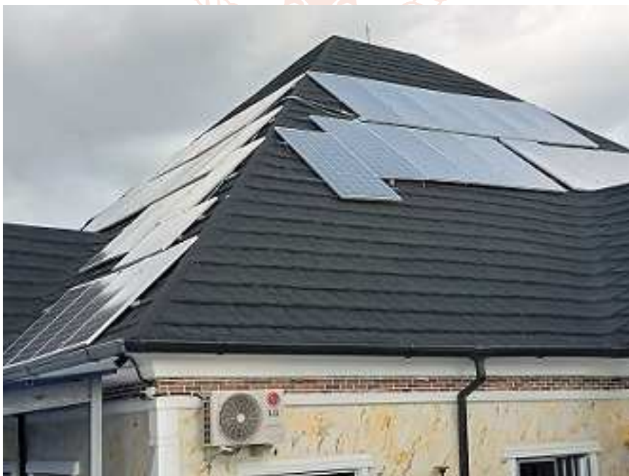
Plate 3: Solar Installation Final
