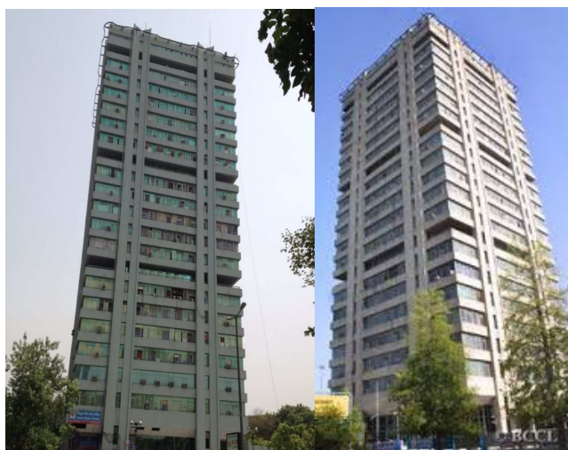
Fig 9 Pic of Vikash Minar for Retro-fit Building
