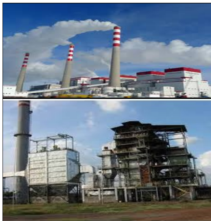
Figure 1: Vardhman Thermal Power Plants
