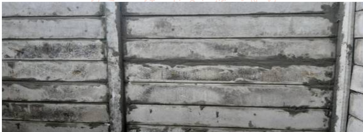
Finishing work in precast construction
