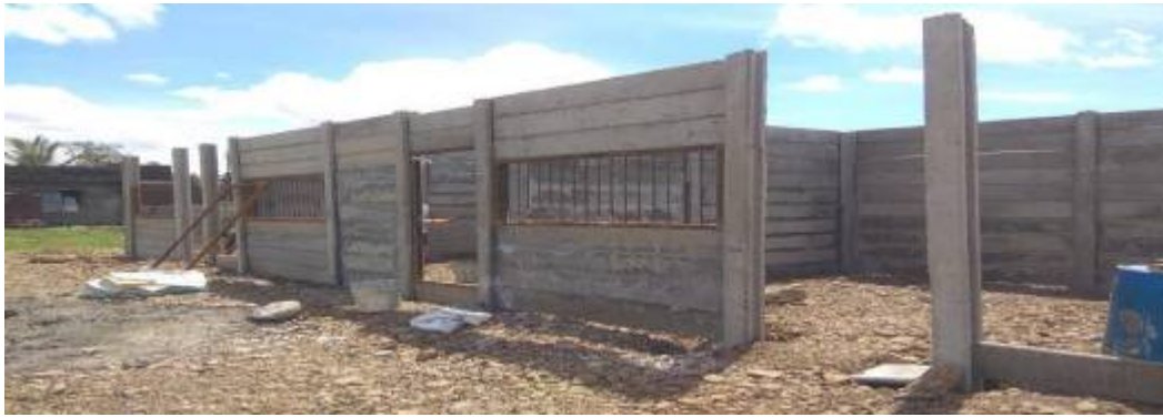
Construction of precast home
