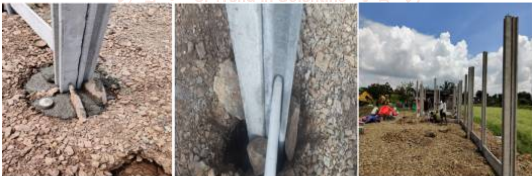
Foundation work in precast construction
