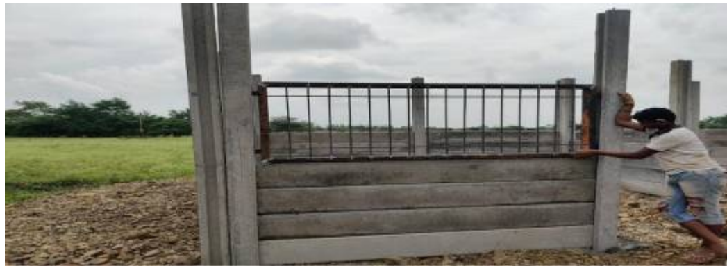
Window fitting between two column
