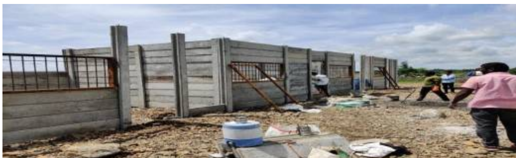
Construction of precast home
