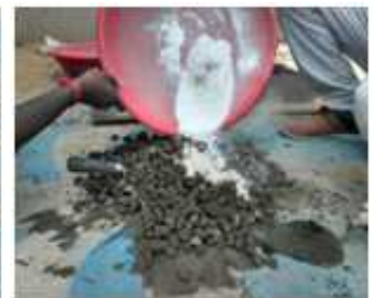
Fig 4.2 Mixing of materials
