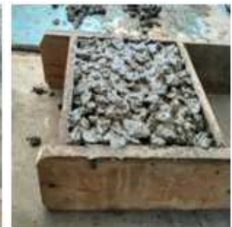
Fig 4.4 Placing of concrete
