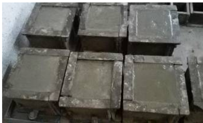
Figure.4.3 Casting of Concrete
