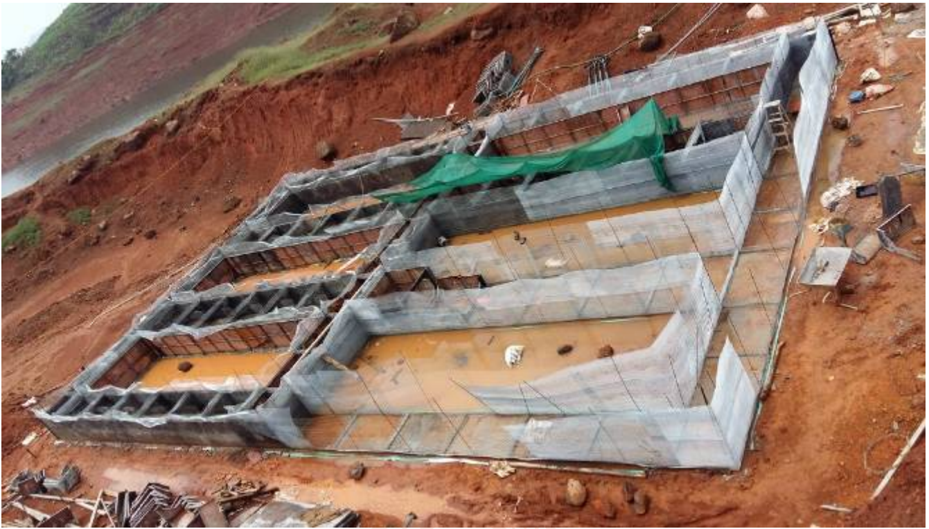
Figure 2: Ferro Cement Platforms
