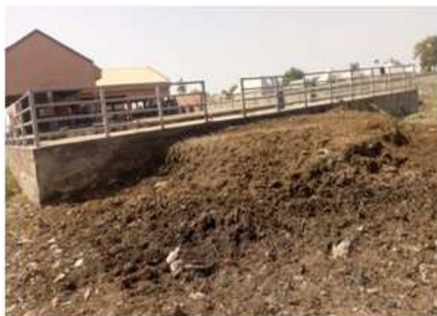
Figure 1 Dumped slaughtered waste at Mubi North SH
