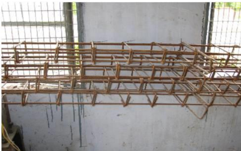
FIGURE 3.7: TENSILE REINFORCEMENT STEEL, WITH HANGER BARS & STIRRUPS
