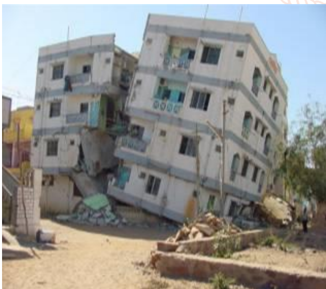
Figure 3 Collapse of the earthquake related failure
