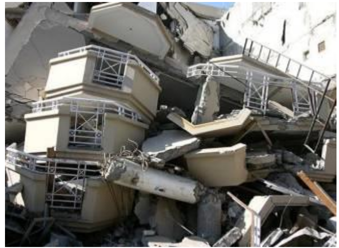
Figure 4. A total Collapse of a Building
