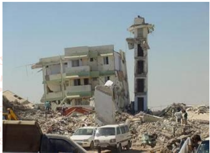
Fig. 5. Apartment collapse in bhuj (2001) Source: www.news.cn
