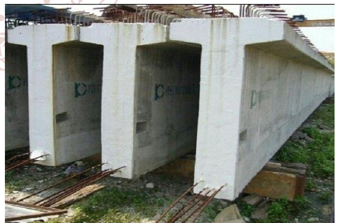
Figure 1 T-Beam Crosssection View
