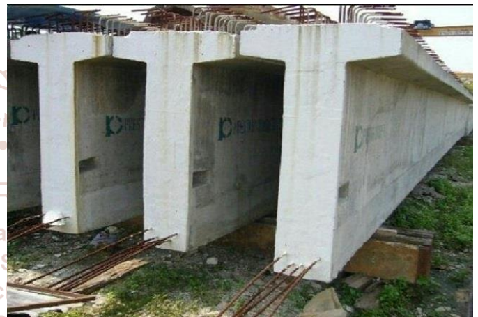
Figure 2. T-Beam Crosssection View
