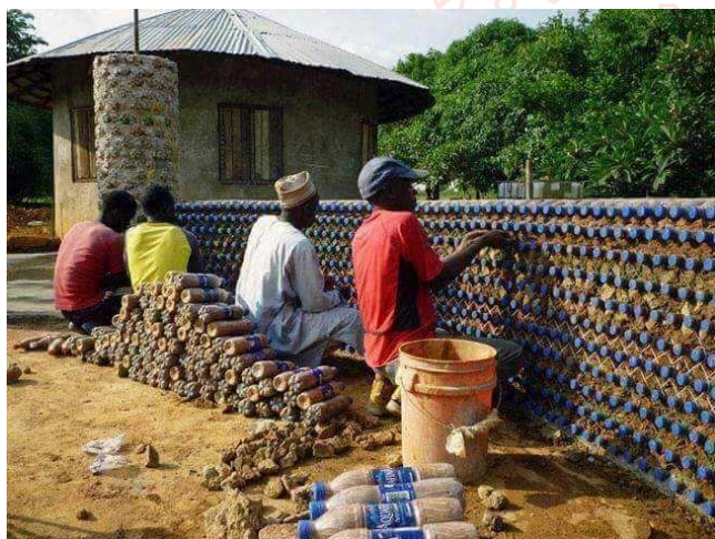
Plate 9. Typical urban poor shelter made of plastic bottles filled with sand.
