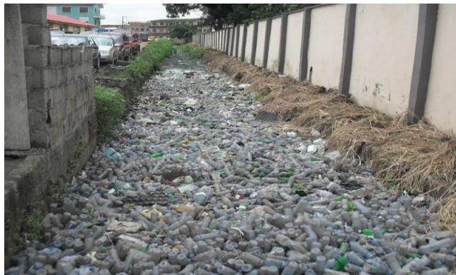
Plate 1. Randle Street, Surulere, Lagos Water Channel clogged with empty plastic water containers Source: Obiadi (2012)
