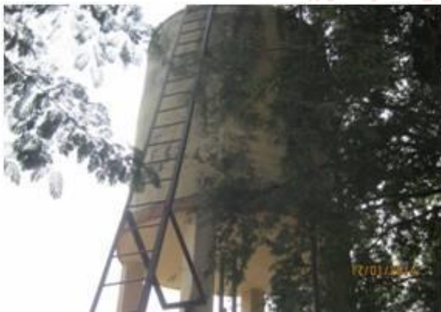
Fig.3.1 Image of the Water Tank
