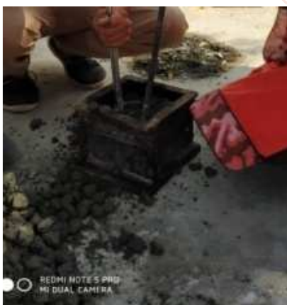
Fig 3.3 Compaction of concrete
