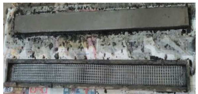
Fig.4.4 Casting of ferrocement laminate
