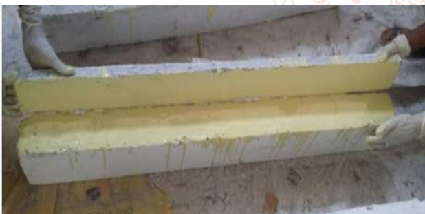
Fig. 4.5 Application of epoxy resin on RC beams and laminates
