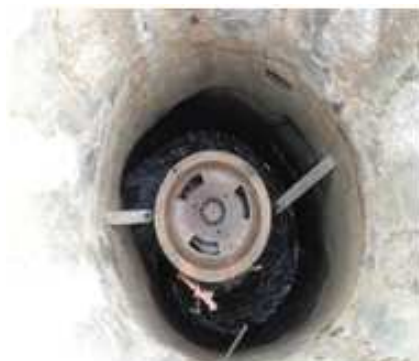
Fig.9. Top View of Generator in Spiral casing
