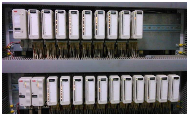
Image of DCS Hardware
