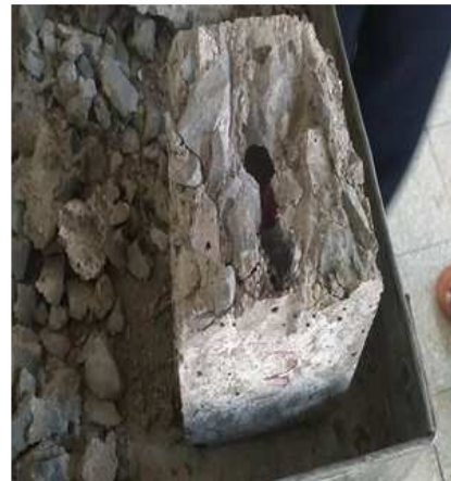
Fig7 Result of carbonation test
