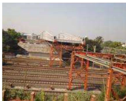
Figure 10 Rolling of leading end girder over trestle (T1)
