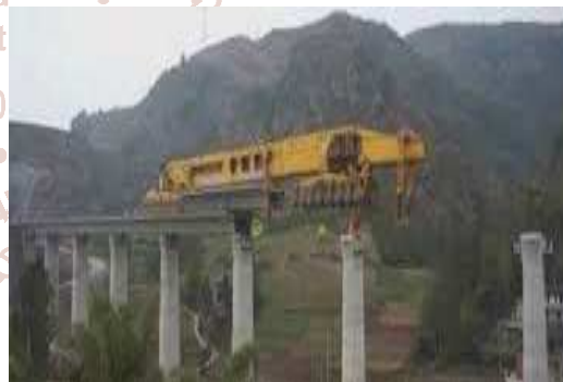
Figure 1 Incremental Launching on site
