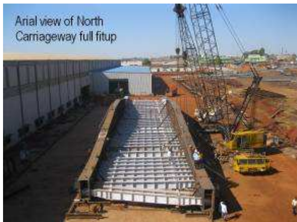
Figure 3 Fabrication work at workshop
