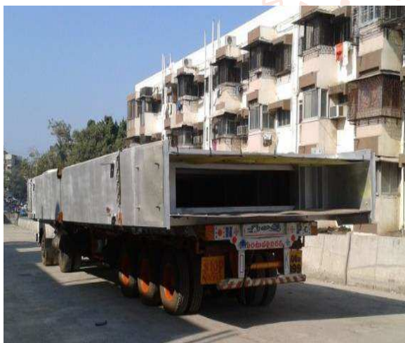
Figure 4 Transportation of carriage way
