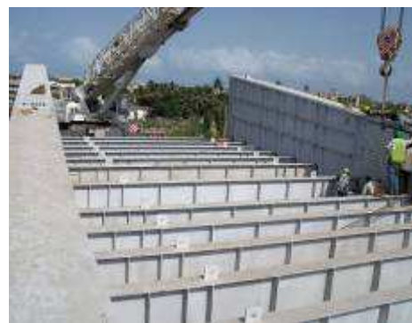
Figure 7 Assembly of second pair of segments – (N2/S2)
