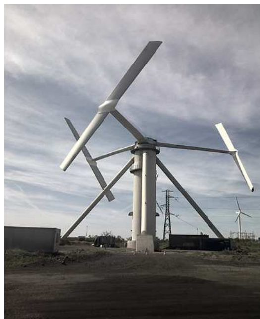
Fig.4- Vertical axis wind turbine
