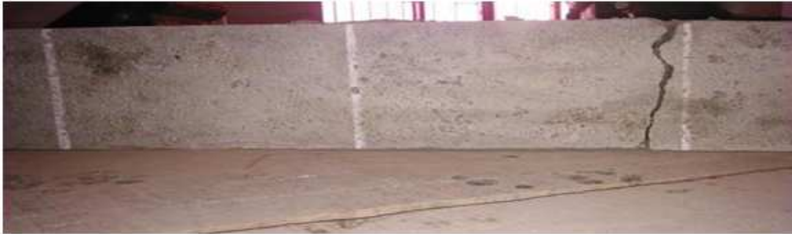
Crack Pattern of P-SC.
