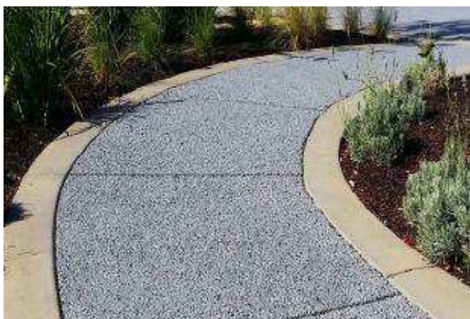
Figure2. Pervious concrete application in sidewalks
