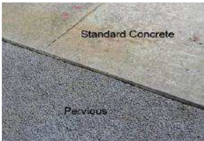
Figure1. Comparison of pervious and conventional concrete
