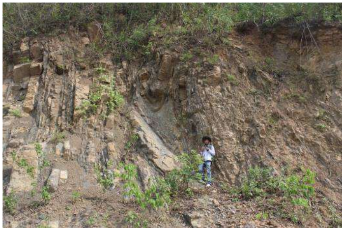
Figure(16) Debris flow of landslide in Loi-an Group (N20° 43' 30"E96° 23' 18")
