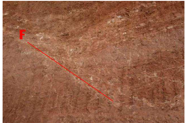
Figure (6) Fault observed at the road cut of the right bank.
