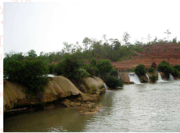
Figure (3.2) Calcareous tufa in river section of dam site
