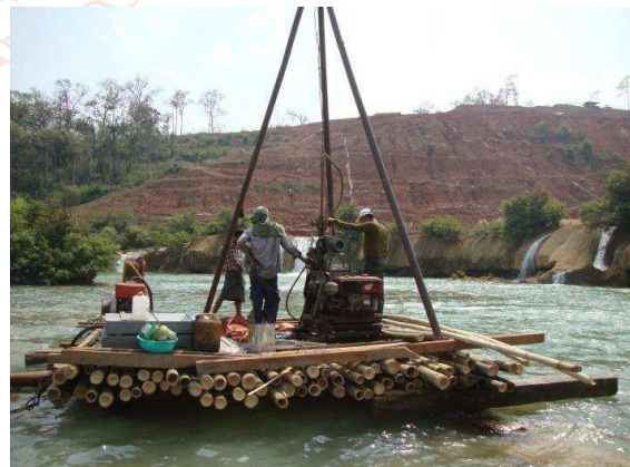
Figure (3.3) ADD 20 working photo at river section
