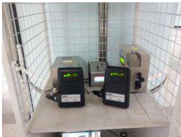
Fig.2. The PM measuring instrument Airstest PM2500 installed at a subway station
