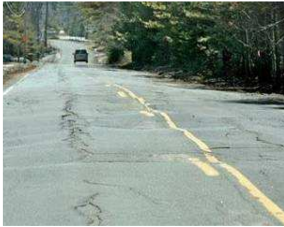
Fig.2 Undulated pavement
