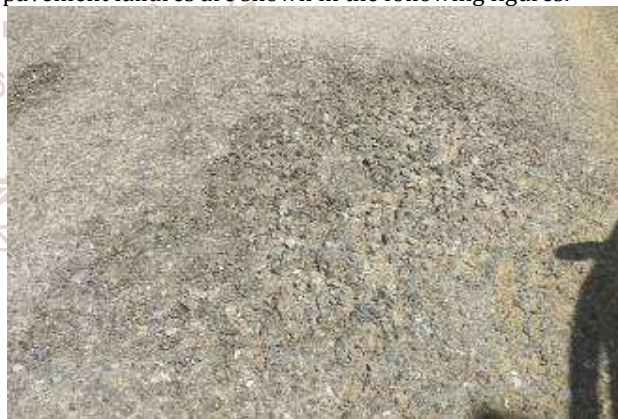
Figure3. Localized Raveling in Tada U Airport Road
