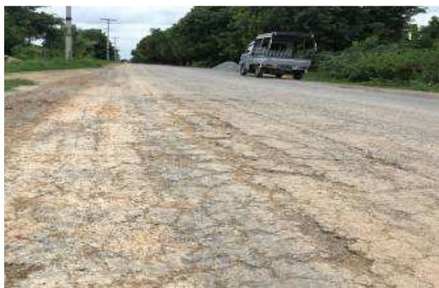
Figure12. Localized Map Cracking in PaleikTada U Road
