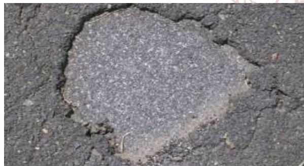
Figure8. Localized Delamination in Tada UAirport Road
