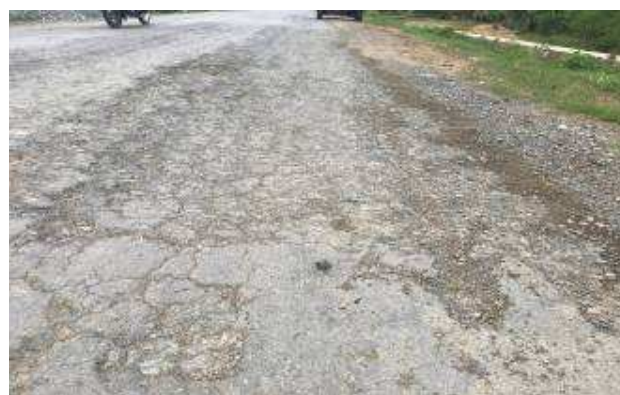
Figure11. Localized Raveling in PaleikTada U Road
