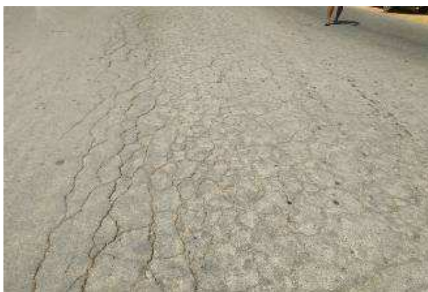
Figure4. Localized Map Cracking in Tada U Airport Road
