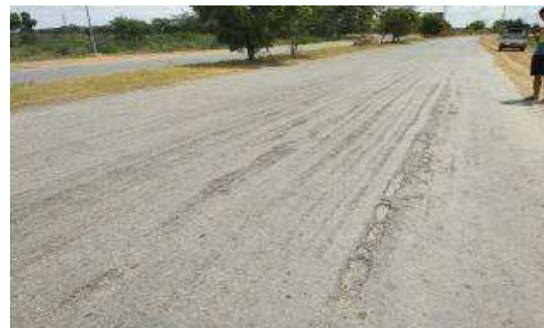
Figure9. Localized Rutting in Tada UAirport Road
