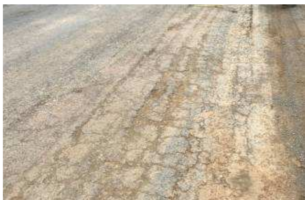
Figure13. Localized Crocodile Cracking in PaleikTada U Road
