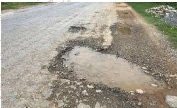
Figure17. Localized Edge Failure in PaleikTada U Road
