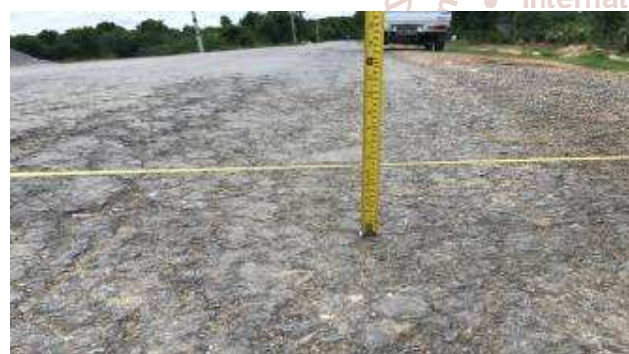
Figure14. Localized Depression in PaleikTada U Road
