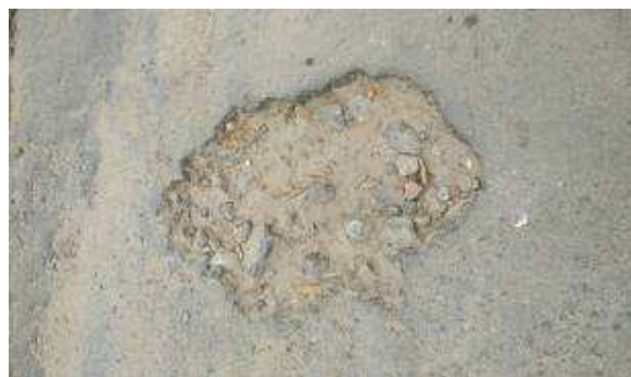
Figure6. Localized Pothole in Tada UAirport Road
