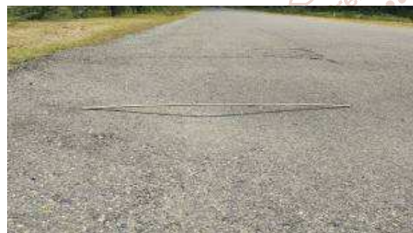
Figure7. Localized Depression in Tada UAirport Road
