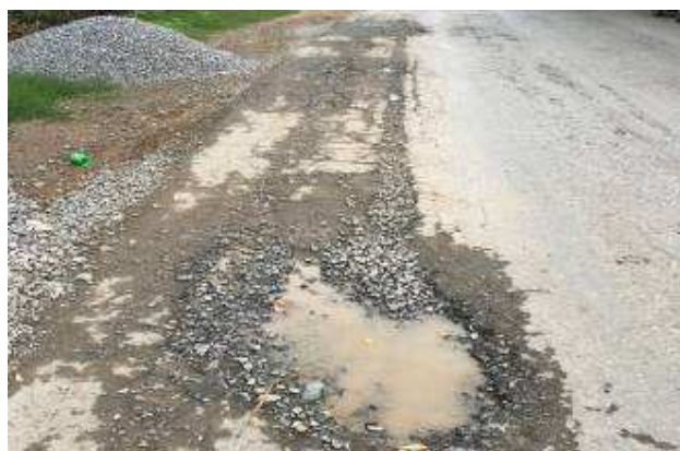
Figure15. Localized Pothole in PaleikTada U Road
