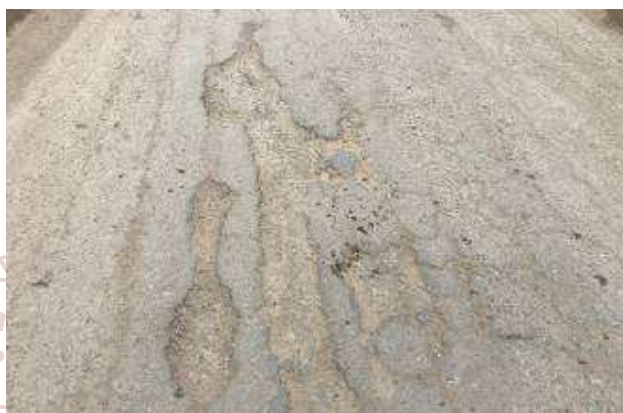
Figure16. Localized Delamination in PaleikTada U Road
