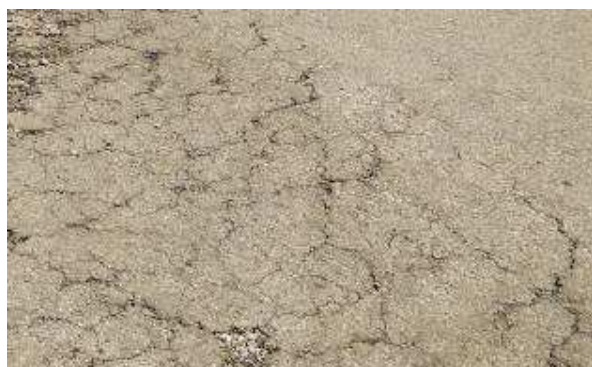
Figure5. Localized Crocodile Cracking in Tada UAirport Road
