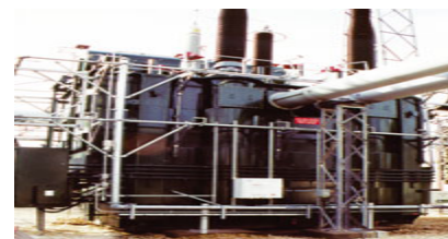
Figure8 - Fiber optic temperature sensor on a 107MVA converter transformer
