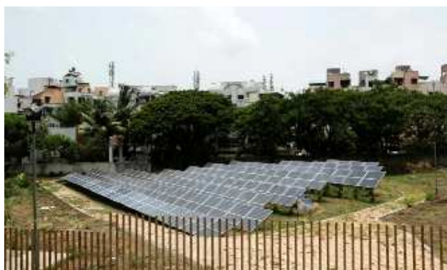
Figure No. 5: 100 Kw Solar PV system
