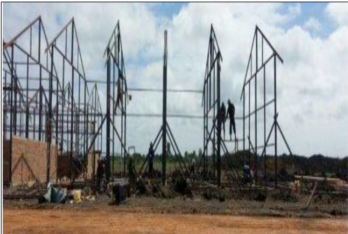
Figure 2: Picture of A Semi-Permanent House That Uses Steel
