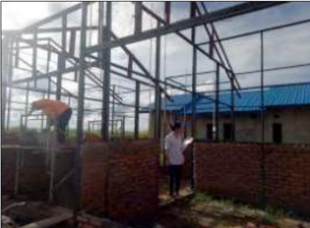
Figure 3: Picture of The Process of Making roof In A Semi-Permanent House Using Steel
