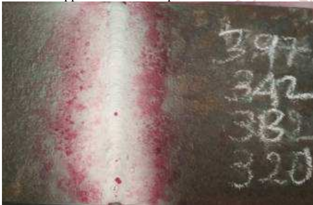
Fig 8: Defects on face layer
