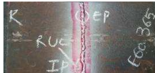
Fig 12: Identifying the defects for E6010 on root layer
