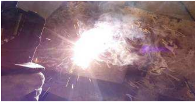
Fig 4: Welding the work piece with E7018
