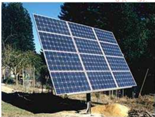
Fig1. Mounted tracking solar array
